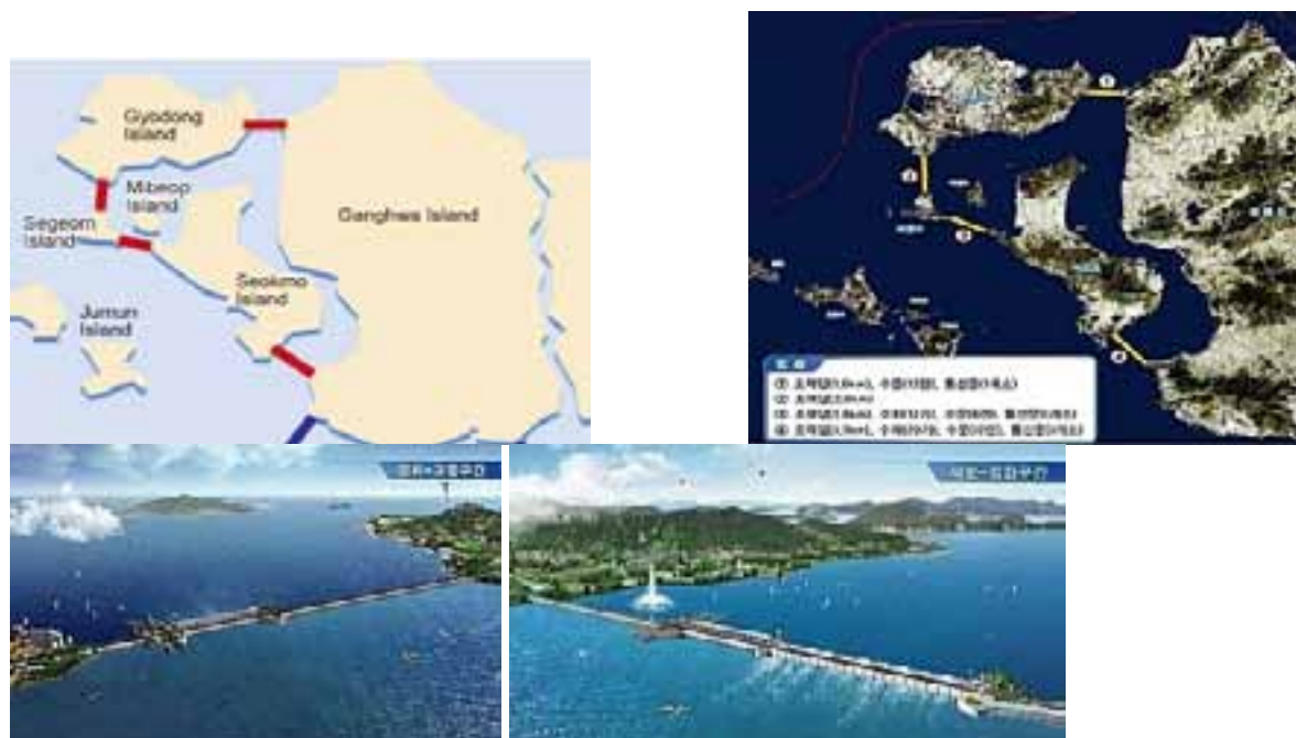
Figure 32: Ganghwa tidal power plant 56
