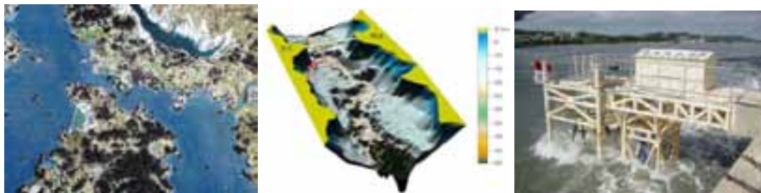
Figure 28: Uldolmok Tidal Current Power Plant (1 MW, experimental) 45
